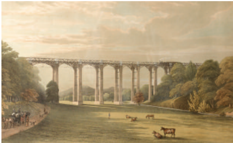
A railway viaduct in South Devon (National Trust).
