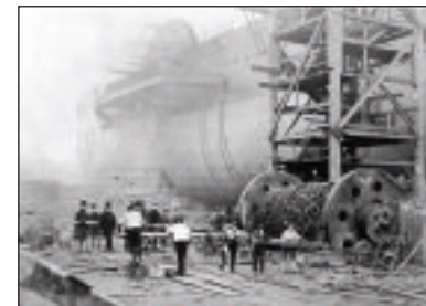
ss Great Eastern during construction (Institution of Civil Engineers).
