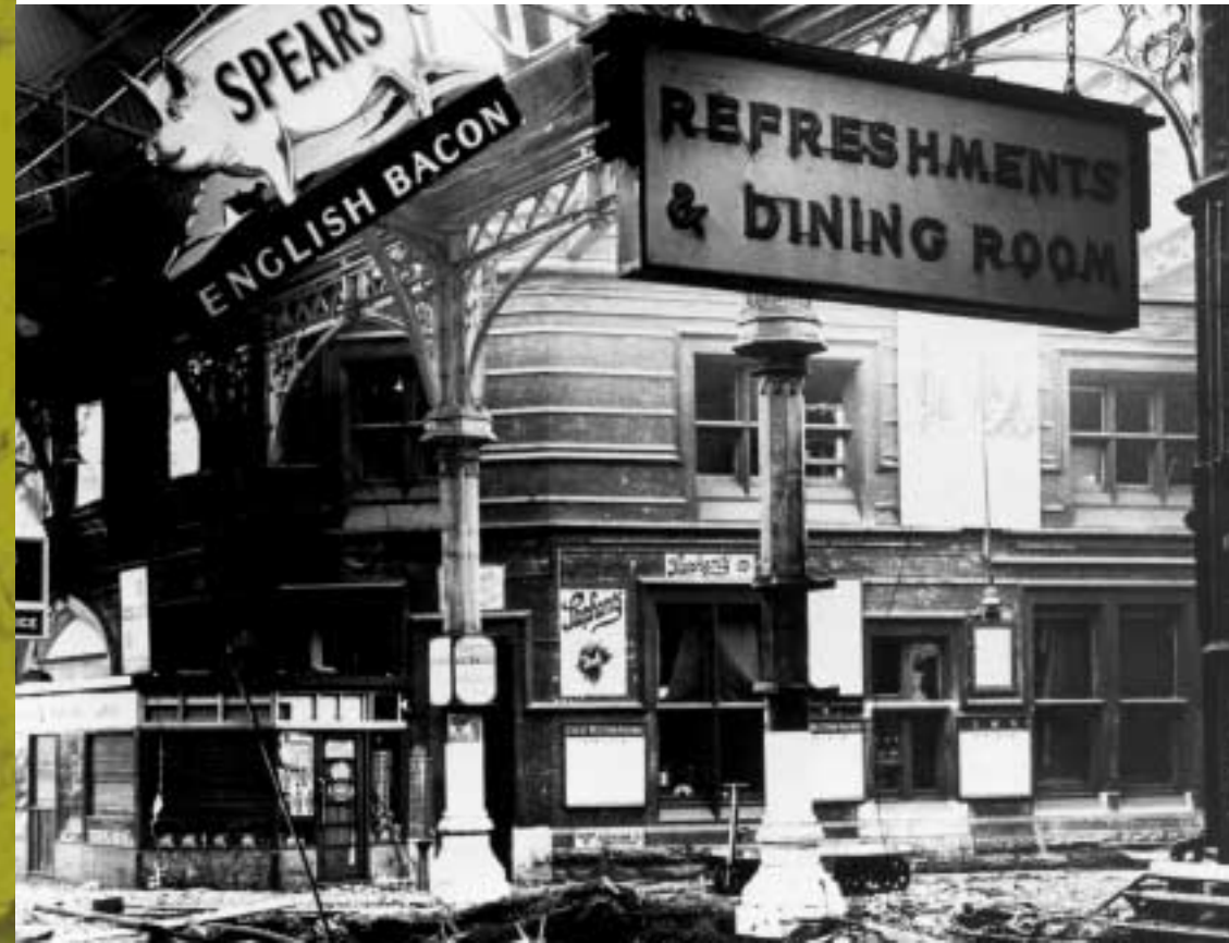
Bomb damage Temple Meads, November 1940
